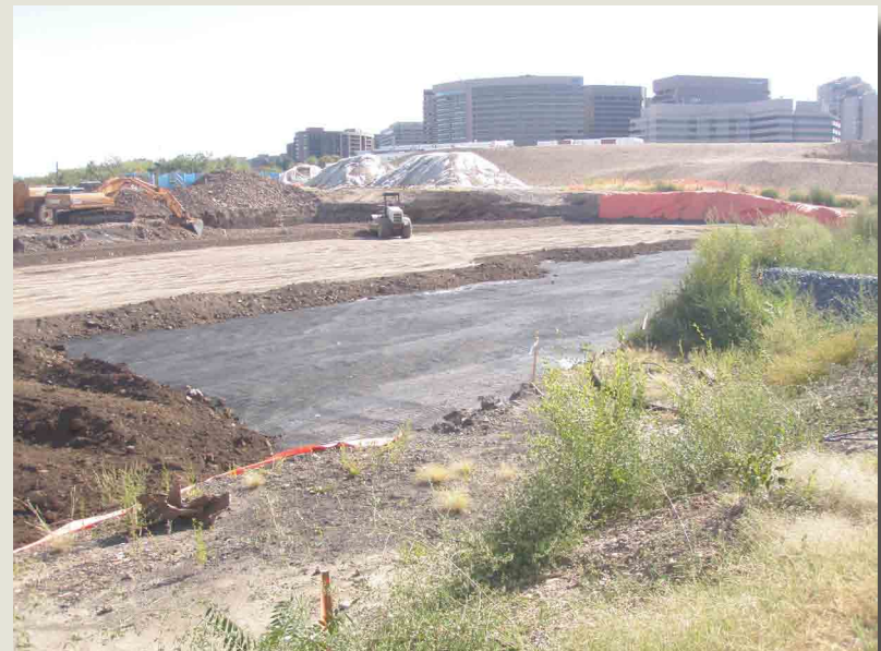
Clean Fill being Placed on the Asphalt Cap, Parcel 14
