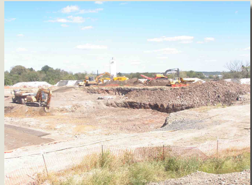
Excavation of Contaminated Soils, Parcel 15
