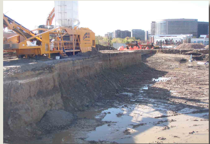
Excavation of Contaminated Soils and Treatment Facility, Parcel 15
