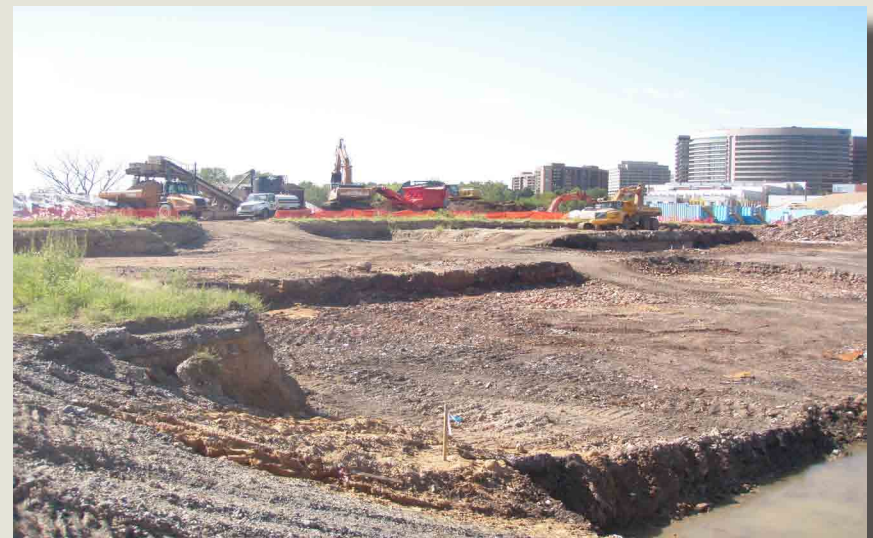
Excavation of Contaminated Soils and Treatment Facility, Parcel 15
